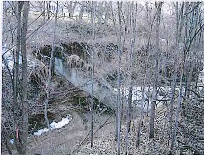
PHOTO 1: This 2011 photo shows the massive washout below the existing grade control structure and how water is being forced below the structure and along the bank. With further degradation, the vertical slopes may encroach on the sanitary outfall sewer located along the channel's south side.
