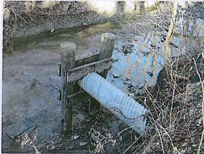
Photo 4. This 2011 photo shows an existing 18" CMP and pile bent structure exposed in the channel. The end of the CMP and pile bent structure were originally constructed at the edge of the channel bank. This photo shows how the channel has eroded approximately 10 feet wider behind the pile bent structure and 6 feet deeper than when originally installed.
