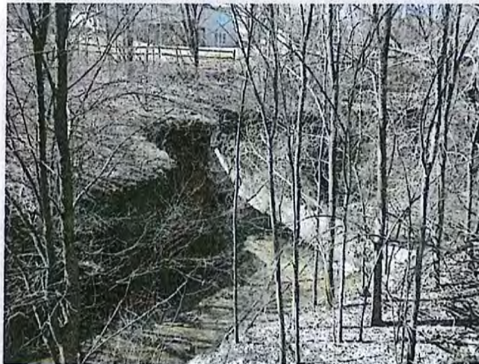
PHOTO 1: This 2011 photo shows the massive washout below the existing grade control structure and how water is being forced below the structure and along the bank. With further degradation, the vertical slopes may encroach on the sanitary outfall sewer located along the channel's south side.
