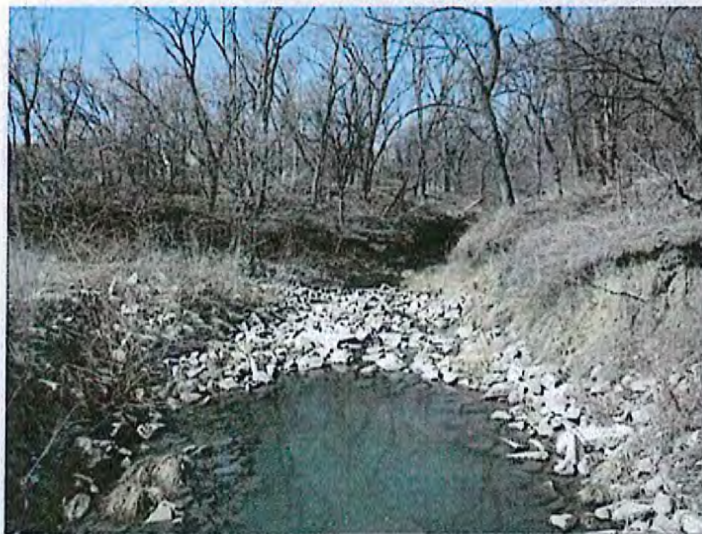
Photo 3A. This 2013 photo taken from the same location shows there has been additional bank erosion and transport of rip rap.
