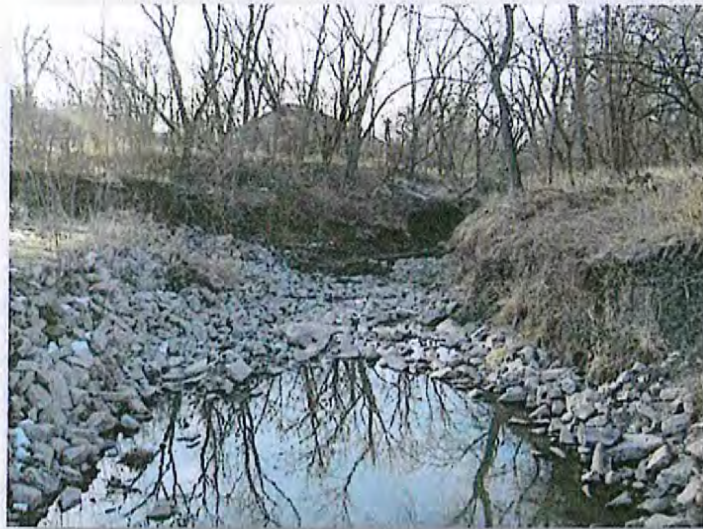
Photo 3. This 2011 photo is taken from standing at the outlet of the 8' x 10' box culvert and the 84" RCP culvert, while looking downstream. The significant washout and erosion along the side slopes can be seen. The large washout of rip rap and movement of rip rap downstream can also be seen in the photo.
